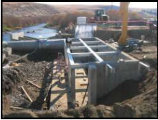
Hofer Dam fish ladder under construction
