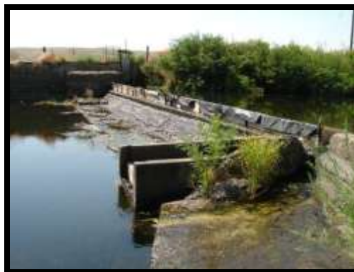
Hofer dam antiquated fish ladder
