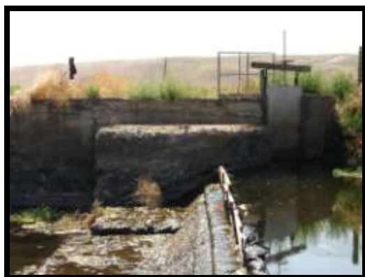
Hofer dam antiquated irrigation diversion
