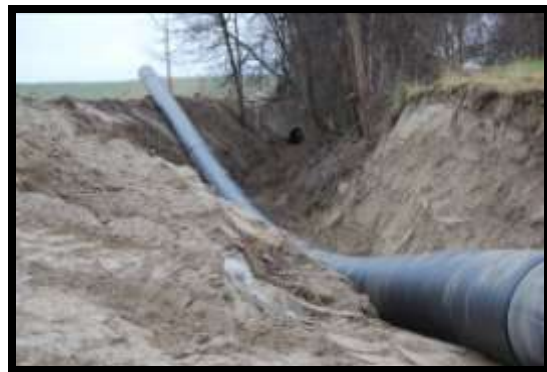
HDPE ready for installation
