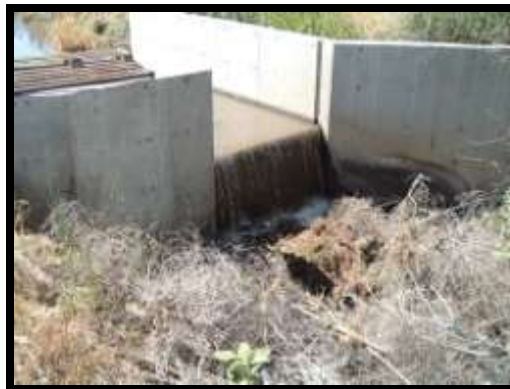
Old structure that splits flow for Westside (60%) and Eastside (40%)
