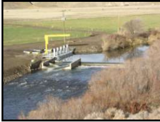
Hofer dam with new fish ladder
