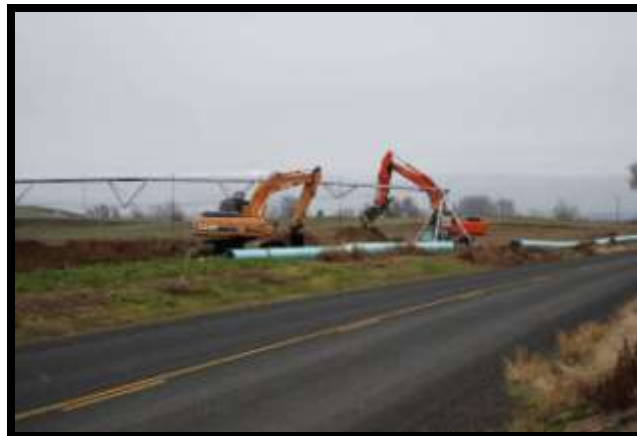
Installation of PVC conveyance line along County road
