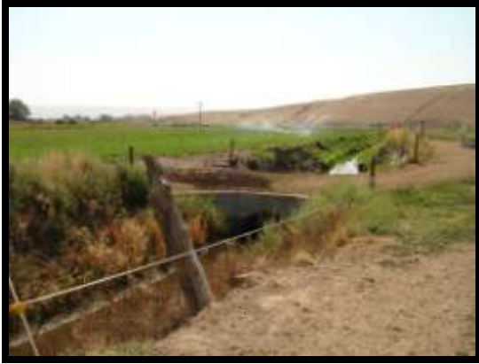
Westside ditch pre-construction
