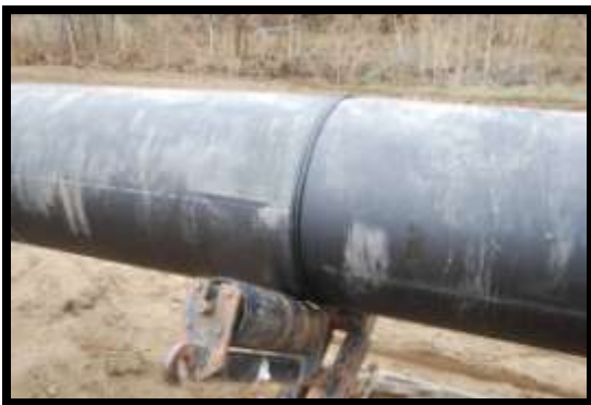
HDPE fusion-welded joint
