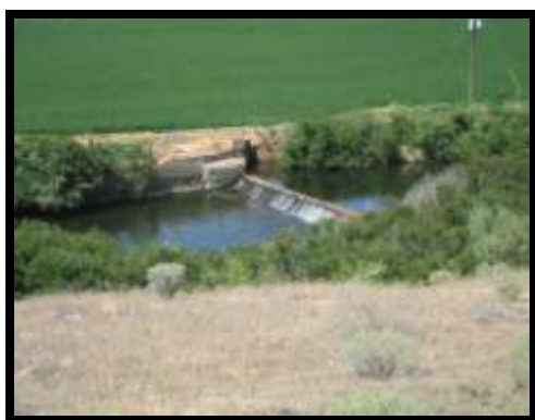
Hofer Dam before remediation
