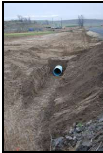
Installed PVC conveyance line
