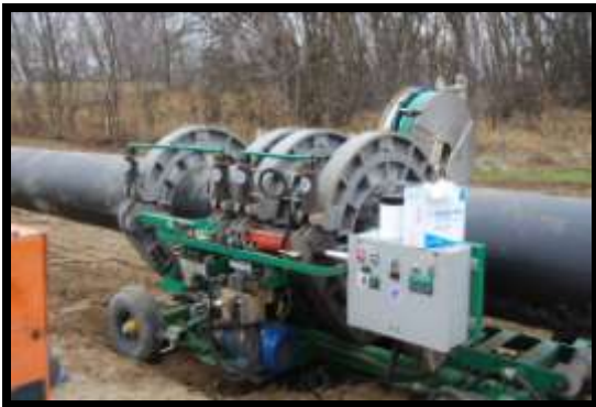
Fusion welding machine that literally melts the sections of pipe together
