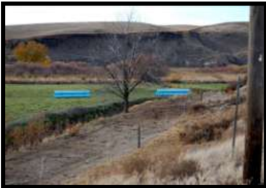
Eastside ditch pre-construction with piping staged
