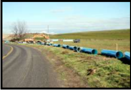
Staged pipe eastside of North Touchet Road
