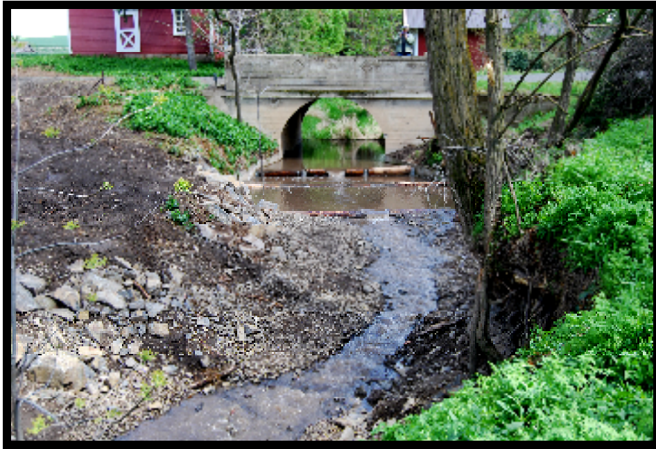
Figure 3: Nowogrowski Farm headquarters bridge looking upstream after the installation of step-up weirs.
