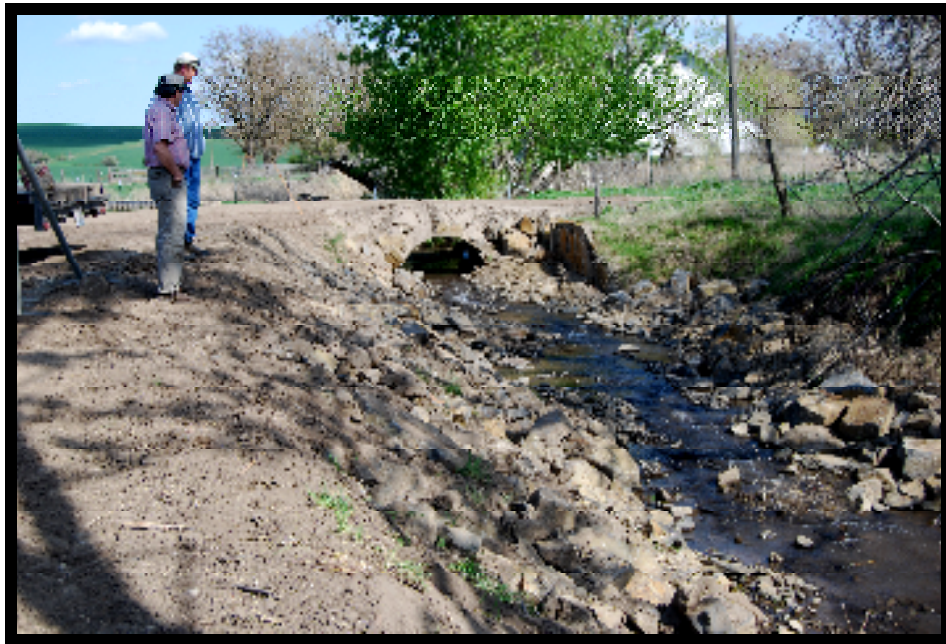
Figure 4: Kibler Farm's new arched culvert after installation of step-up weirs.
