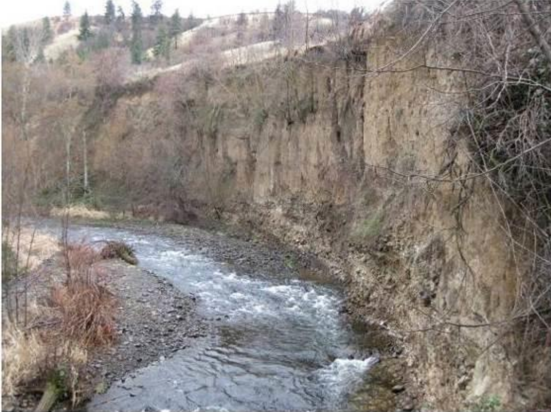
Figure 18. Eroding stream bank just above private bridge at RM 2.7
