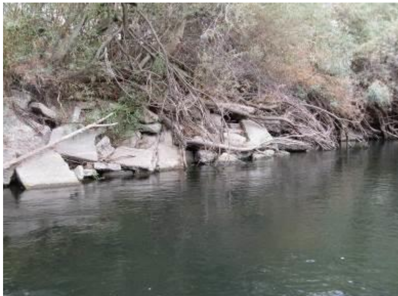
Figure 53. Concrete rip-rap along the channel banks offers little fish habitat; Walla Walla County, Washington
