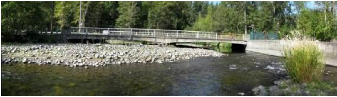
Figure 25. Photo of upstream sediment deposition as a result of flow constriction created by the Wickersham Bridge, Mill Creek, Walla Walla County, Washington
