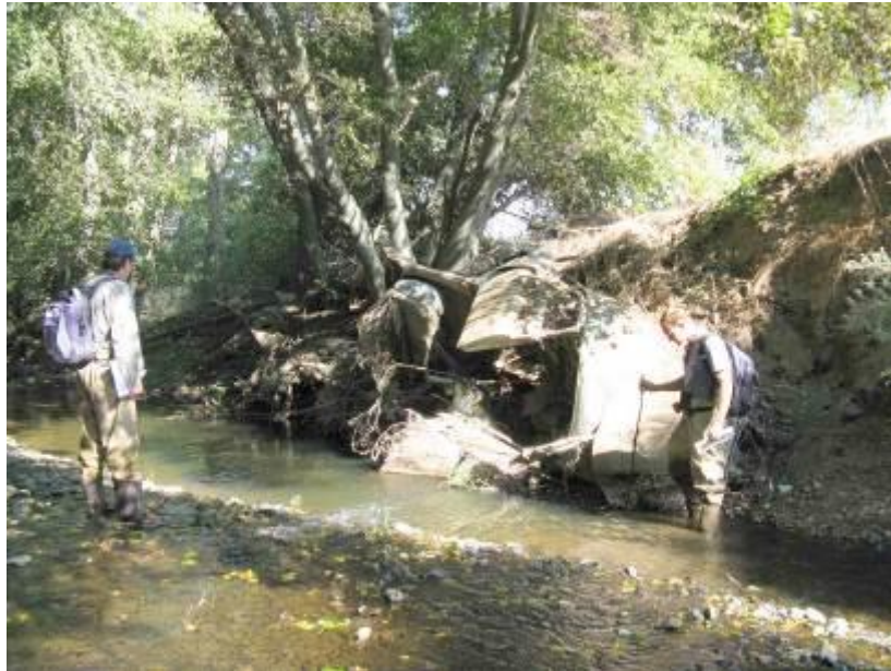
Figure 55. Car body placed in channel presumably to prevent erosion; Walla Walla County, Washington
