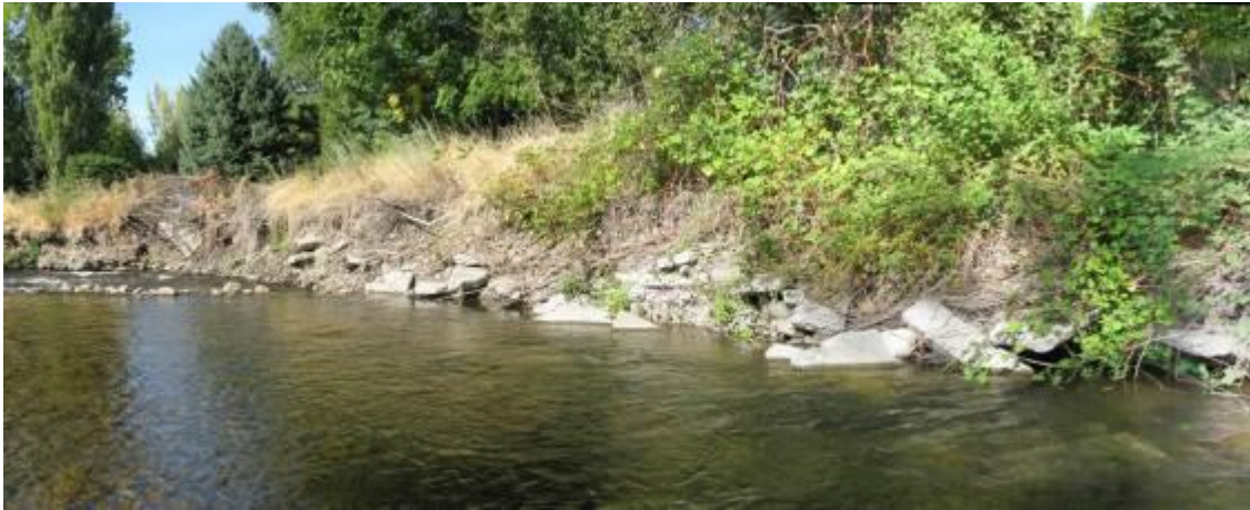
Figure 54. Concrete rip-rap along the channel banks offers little fish habitat; Walla Walla County, Washington
