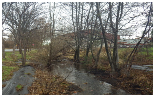
After: Weeds and debris removed. Plantings are scheduled in spring.
