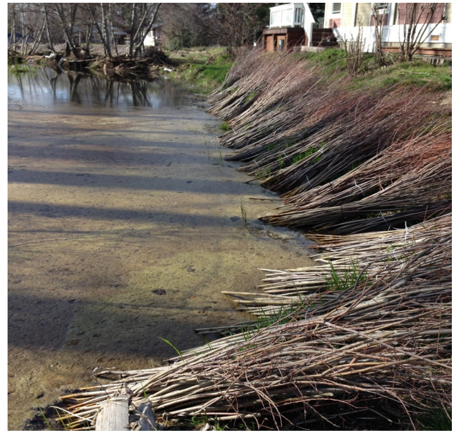
3000 willow whips were harvested and soaked (as shown above) for planting on a section of creek stripped of vegetation by the Feb. 2020 flood. It will take years for nature to regrow the lost trees and shrubs. Landowners can kick start regrowth by planting this fall. Contact Renee if you are interested. We are planning projects for fall and spring.
