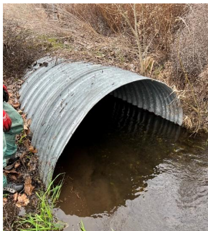
Figure 3. Culvert assessed by WWCCD staff.
