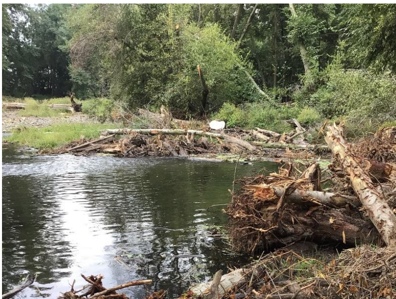
Figure 7: Stream restoration structures on the Walla Walla River
