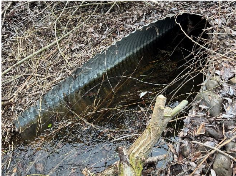
Figure 9: Culvert assessed by WWCCD staff
