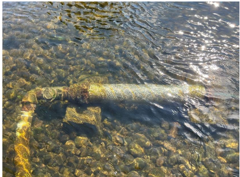
Figure 5: An old fish screen that WWCCD helped to replace using VSP funds
