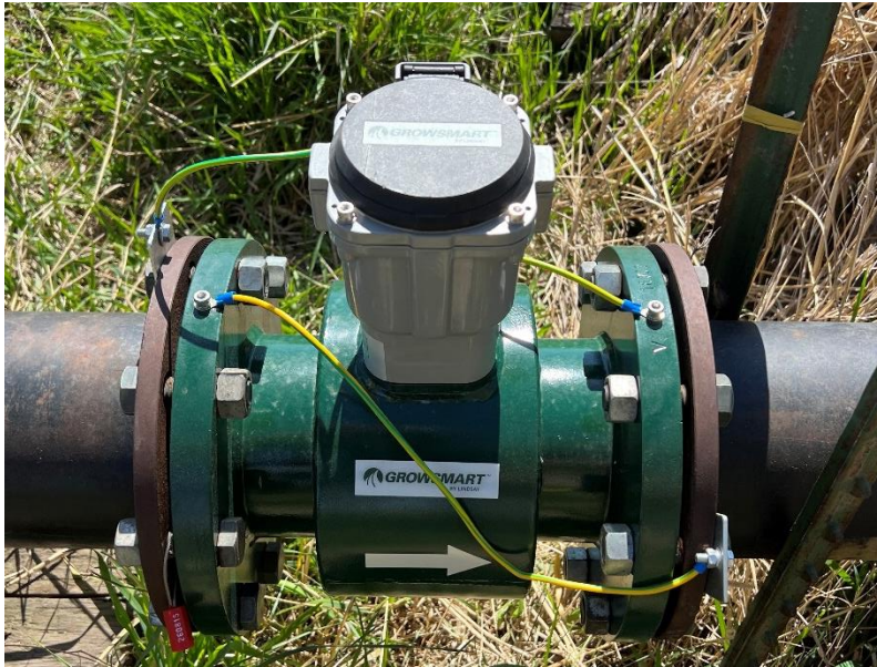
Figure 22: New irrigation flow meter that WWCCD helped a landowner obtain with VSP funds
