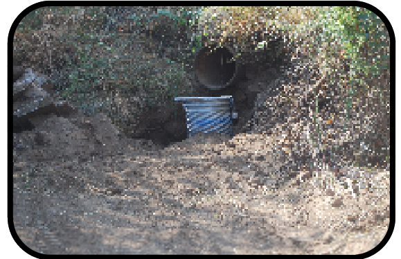
NEW PIPELINE INTAKE STRUCTURE
