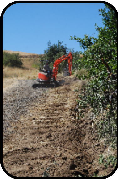
BACKFILLING PIPELINE TRENCH
