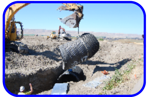
ANGLED PIPE SECTION INSTALLATION
