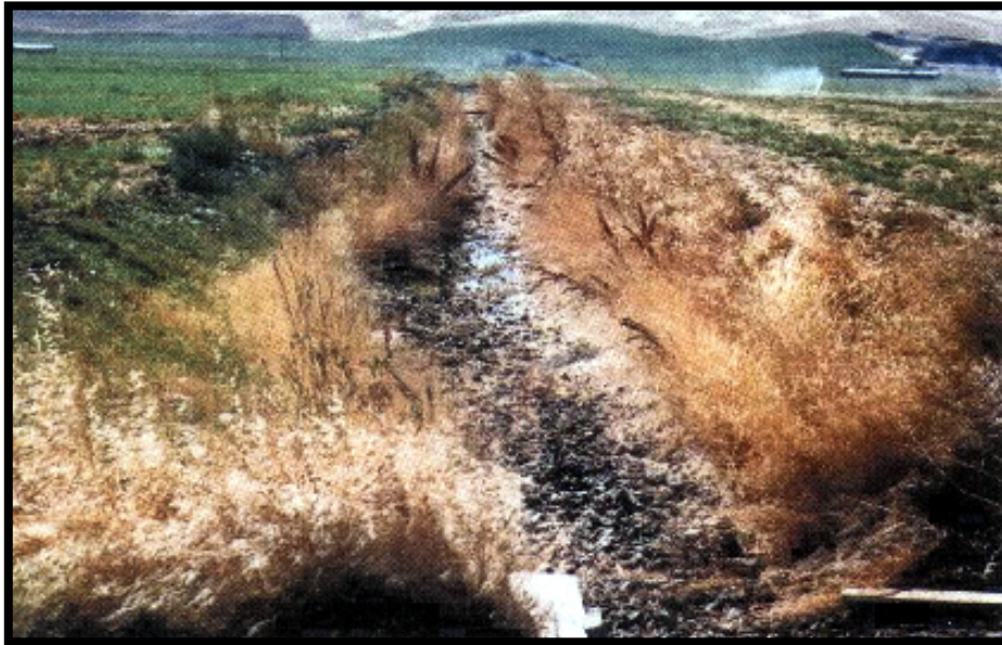
The Riggs Lateral prior to the project. Infiltration and evaporation losses were very high with an open ditch in an arid region.
