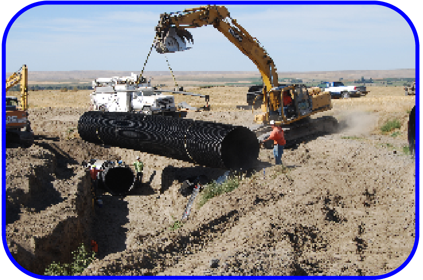
2,800 FT. PROJECT PIPE PLACEMENT OF A 48-FT. LONG SECTION OF 66-INCH PIPE
