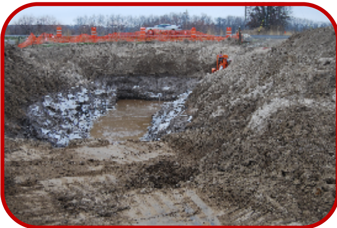
BORE HOLE SITE TO BRING PIPE-LINE UNDER HWY 12
