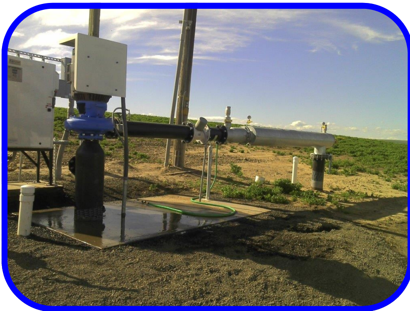
NEW VARIABLE FREQUENCY DRIVE (VFD) PUMP STATION INSTALLATION ON THE GARDENA FARMS IRRIGATION DISTRICT #13 NORTH LATERAL
