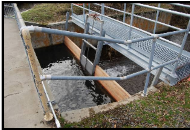
New Garrison Creek headgate downstream of the new screen
