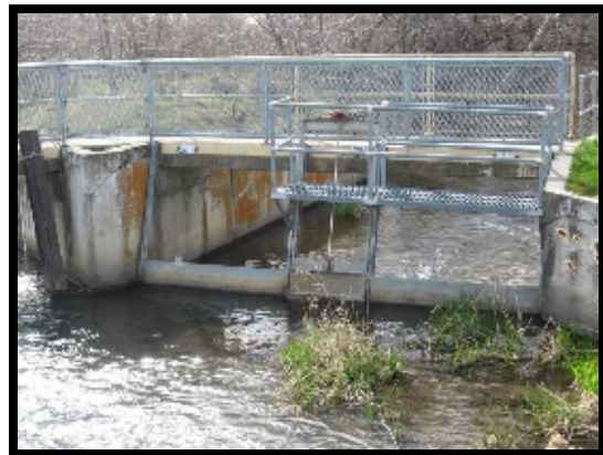
Garrison Creek unscreened headgate Upstream of diversion
