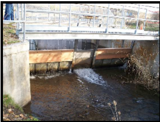
Garrison Creek unscreened headgate downstream of diversion
