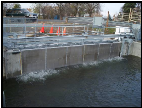
Garrison Creek fish screen bubbler In operation
