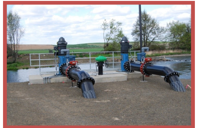
LEFT: PIPELINES COMING FROM NEW PUMPS AT THE DIVERSION STRUCTURE ANCHORED WITH CONCRETE THRUST BLOCKS. RIGHT: NEW 40 HP PUMPS SET TO DELIVER WATER TO THE NEW BWOL PIPED DELIVERY SYSTEM.
