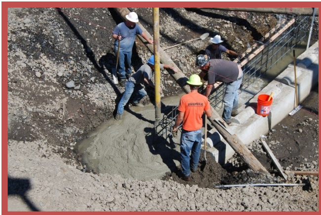
POURING THE BASE PAD AND SETTING INITIAL REBAR WAS DONE IN THE WET. AFTER THE FLOOR WAS POURED, WORK PROGRESSED AT A MORE RAPID PACE.
