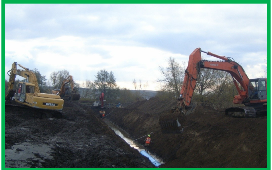
TRENCHING THROUGH VERY WET CONDITIONS
