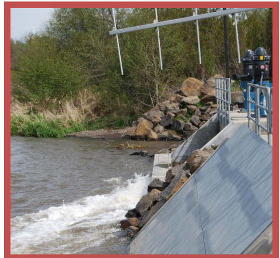
AIR BLAST IN OPERATION CLEANING DEBRIS OFF THE SCREEN
