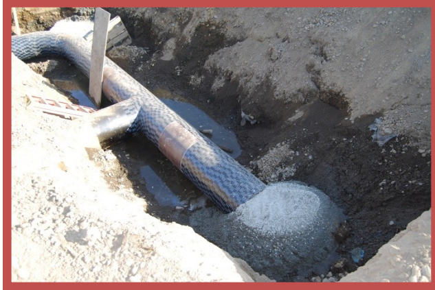
LEFT: PIPELINES COMING FROM NEW PUMPS AT THE DIVERSION STRUCTURE ANCHORED WITH CONCRETE THRUST BLOCKS. RIGHT: NEW 40 HP PUMPS SET TO DELIVER WATER TO THE NEW BWOL PIPED DELIVERY SYSTEM.
