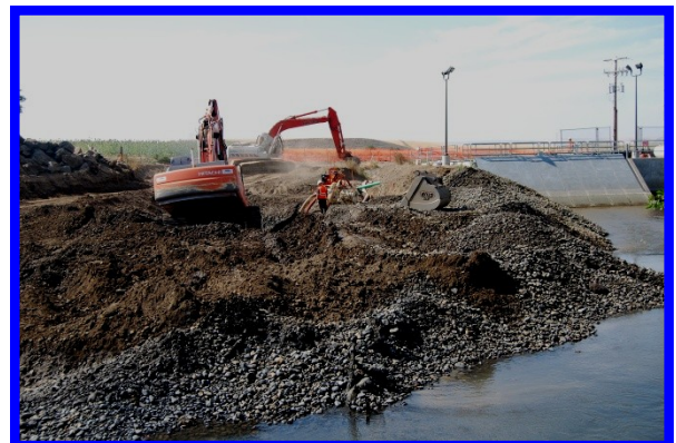
PREPARING STRUCTURE SITE
