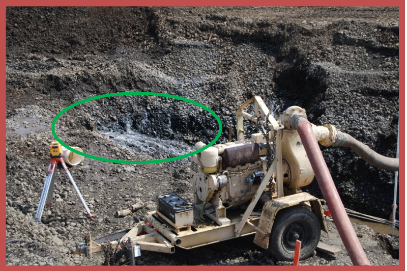
PUMPING EXCESS WATER FROM STRUCTURE SITE. NOTE RAPID SEEPAGE COMING THROUGH GRAVELS.
