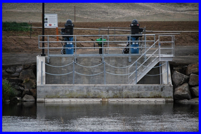
THE COMPLETED BWOL CONSOLIDATED DIVERSION STRUCTURE ON THE WALLA WALLA RIVER
