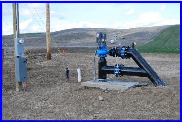
NEW PUMPING STATION
