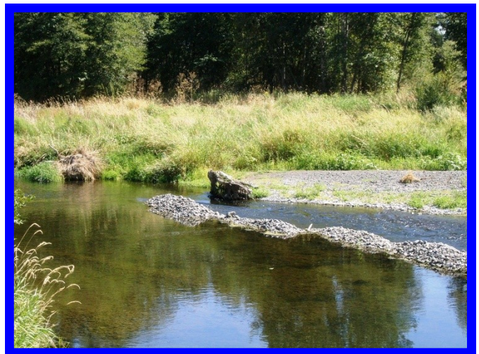
BERGEVIN-WILLIAMS GRAVEL PUSH-UP DAM ON THE WALLA WALLA RIVER NEAR RIVER MILE 31.5
