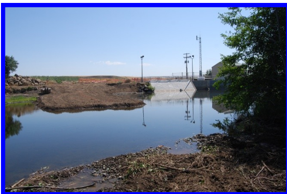
FIRST STAGES OF CONSTRUCTION
