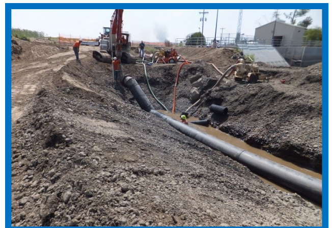
PLACEMENT OF HDPE IN THE TRENCH UNDER THE WALLA WALLA RIVER
