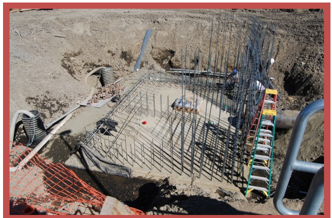
POURING THE BASE PAD AND SETTING INITIAL REBAR WAS DONE IN THE WET. AFTER THE FLOOR WAS POURED, WORK PROGRESSED AT A MORE RAPID PACE.
