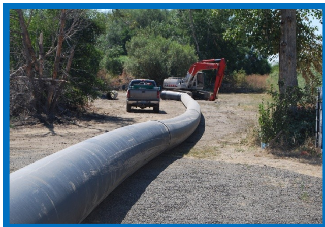
PRE-ASSEMBLED 30-INCH FUSION WELDED HDPE READY FOR PLACEMENT
