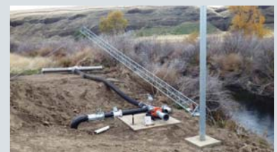
This 500 gallon-per-minute passive fish screen protects endangered fish species during the irrigation season and is ready for launch.
