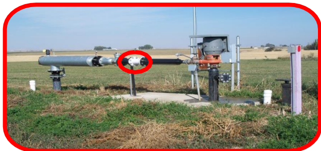
New meter installation
