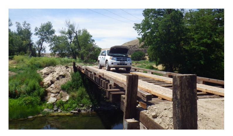
The completed bridge, while not likely to be nominated for most beautiful bridge of the year, allows Gailey to safely access his fields while staying out of the river, reducing bank erosion and sediment delivery to the river. Greg Kinsinger, in taking the final report pictures, looked over the side and saw fish swimming placidly below—a fitting image, highlighting the important results of the conservation work of local farmers.
