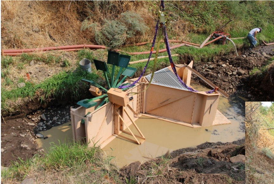
WDFW delivered and helped install the rotating drum screen.
