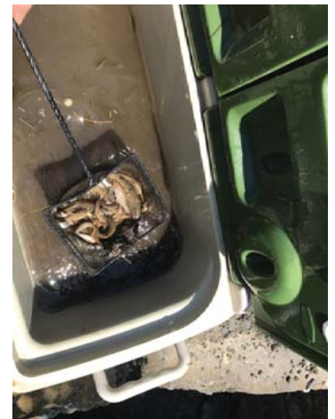
Nearly 200 salmonids and over 300 fresh water fish were salvaged during construction. Photo credit: Sean Taylor, WDFW
