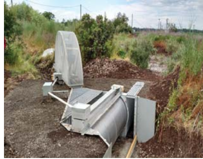
Fish Screen with 6.4 cubic feet per second flow capacity will save lives of salmon. Photo credit: Lisa Stearns, WWCCD
