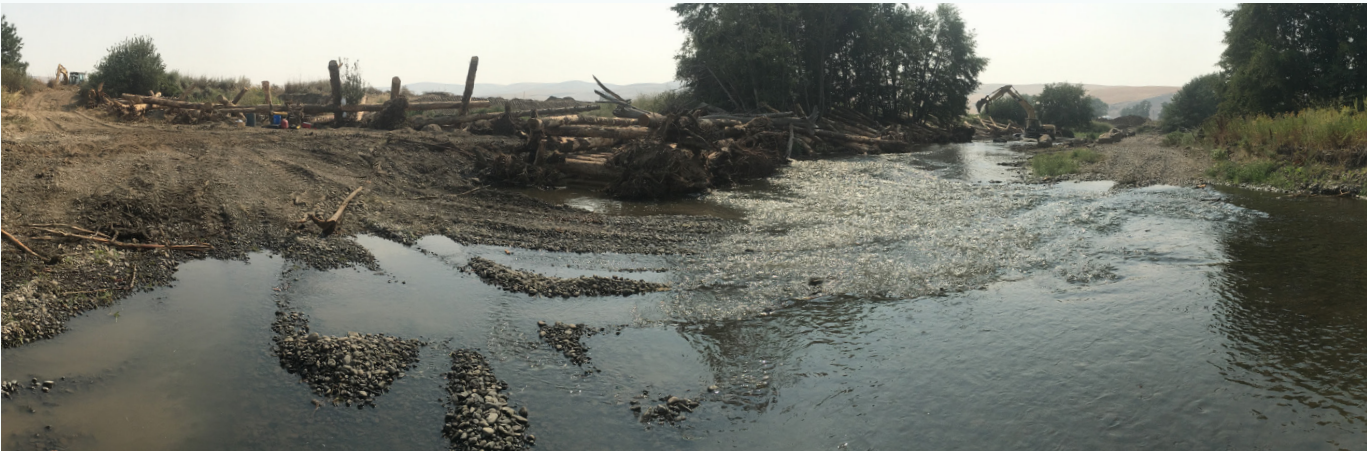
Looking downstream: Pictured left is the Channel Spanning Structure, to the right is the main channel and Multi-log LWD.
