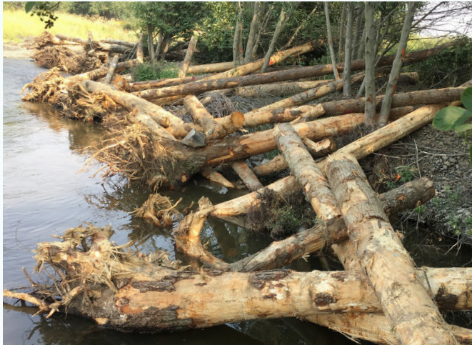
Multi-log LWD along the main channel.
