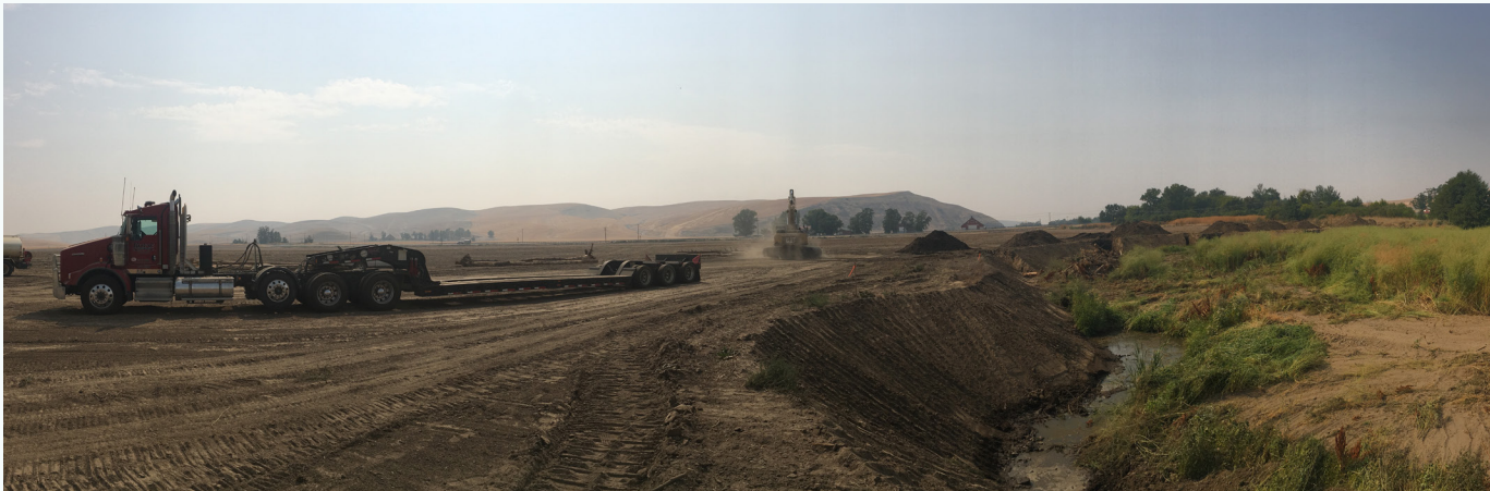
Gravel delivery and bank reshaping.
