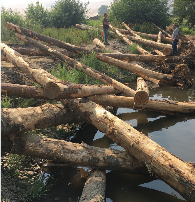
Completed Multi-log LWD before replanting.
