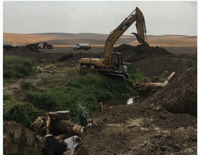
Reshaping the high-water channel.
