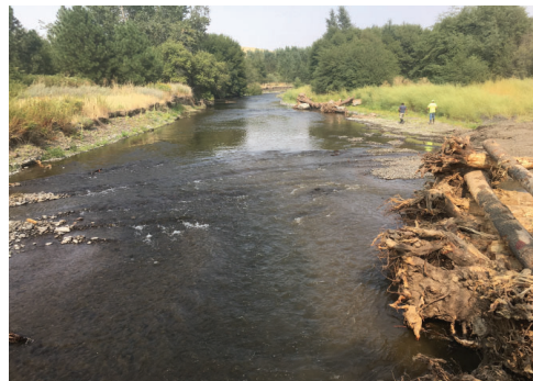
Log structures add habitat components to improve habitat for Endangered Species Act-listed salmon on the Touchet River. Photo credit: Lisa Stearns
