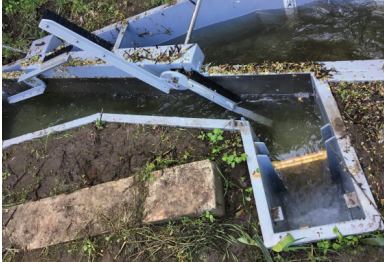
Installed two fish screens on irrigation systems to protect endangered salmon.
